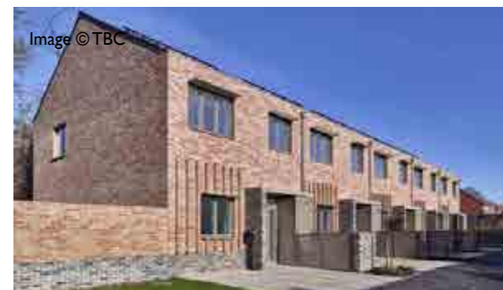
Considered bin enclosure design for terraced housing. Riverside Rd housing, Watford by Bell Phillips
