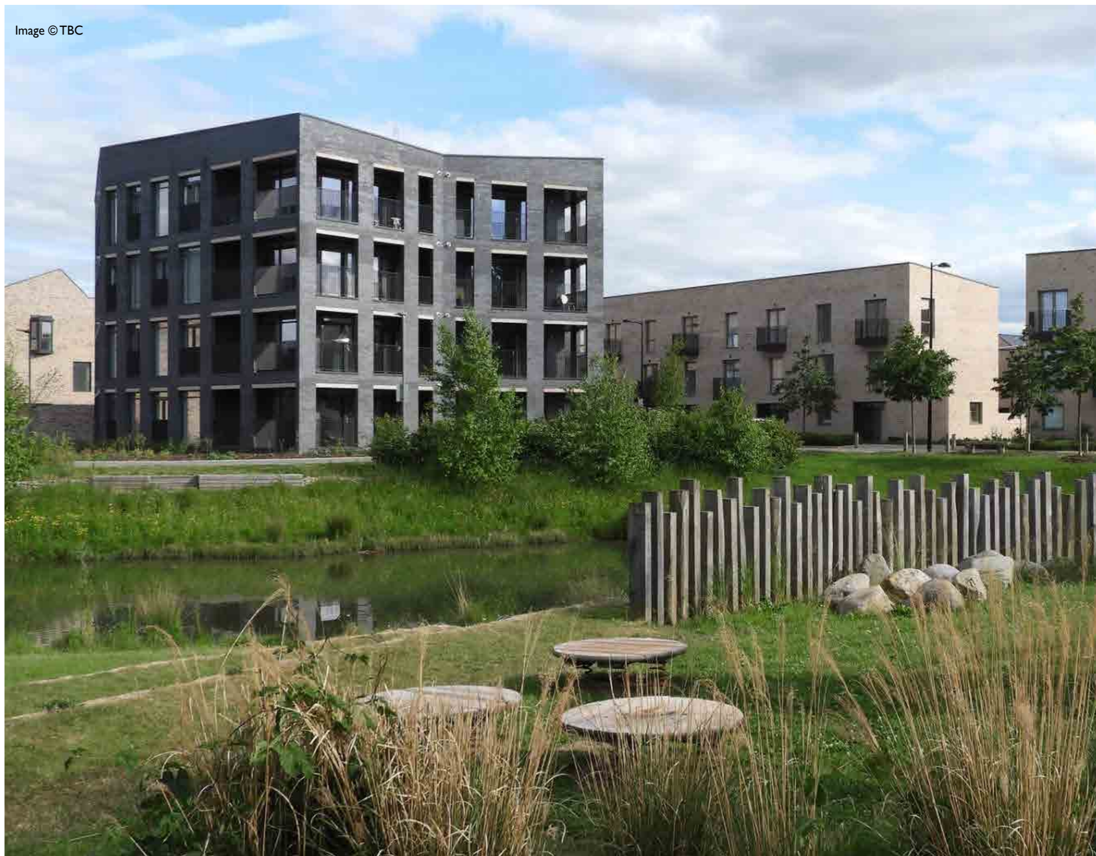
Space for ecology enhancing planting and play around wetlands at Barton Park, Oxford
