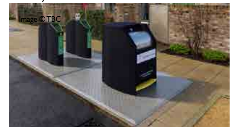
Underground refuse and recycling system
