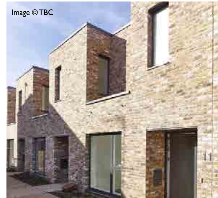
Smaller scale broken terrace Bracelet Close, Corringham, by Bell Phillips Architects
