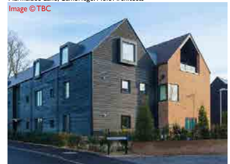
Image © TBC Apartment block form integrated with housing The Avenue, Saffron Walden, by Pollard Thomas Edwards Architects
