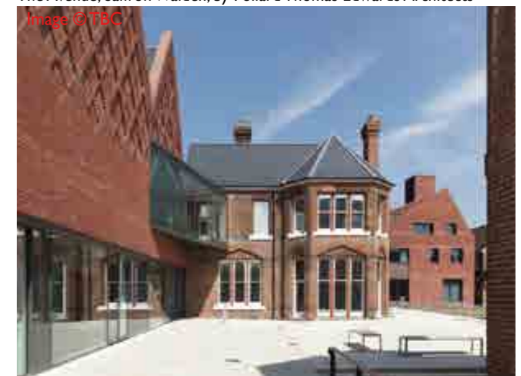
Image © TBC Sensitive school design that promotes activity at Brentwood School by Cottrell & Vermeulen Architects
