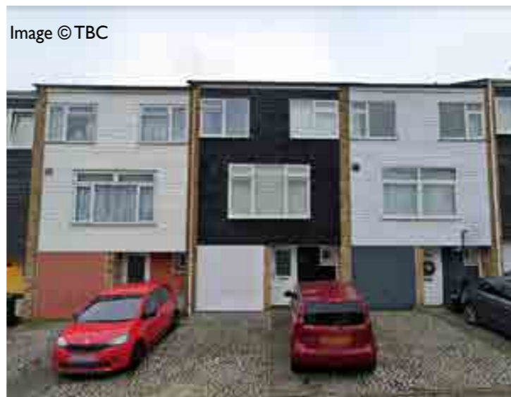
Morley Grove, Little Parndon, Harlow by Gibberd and partners
